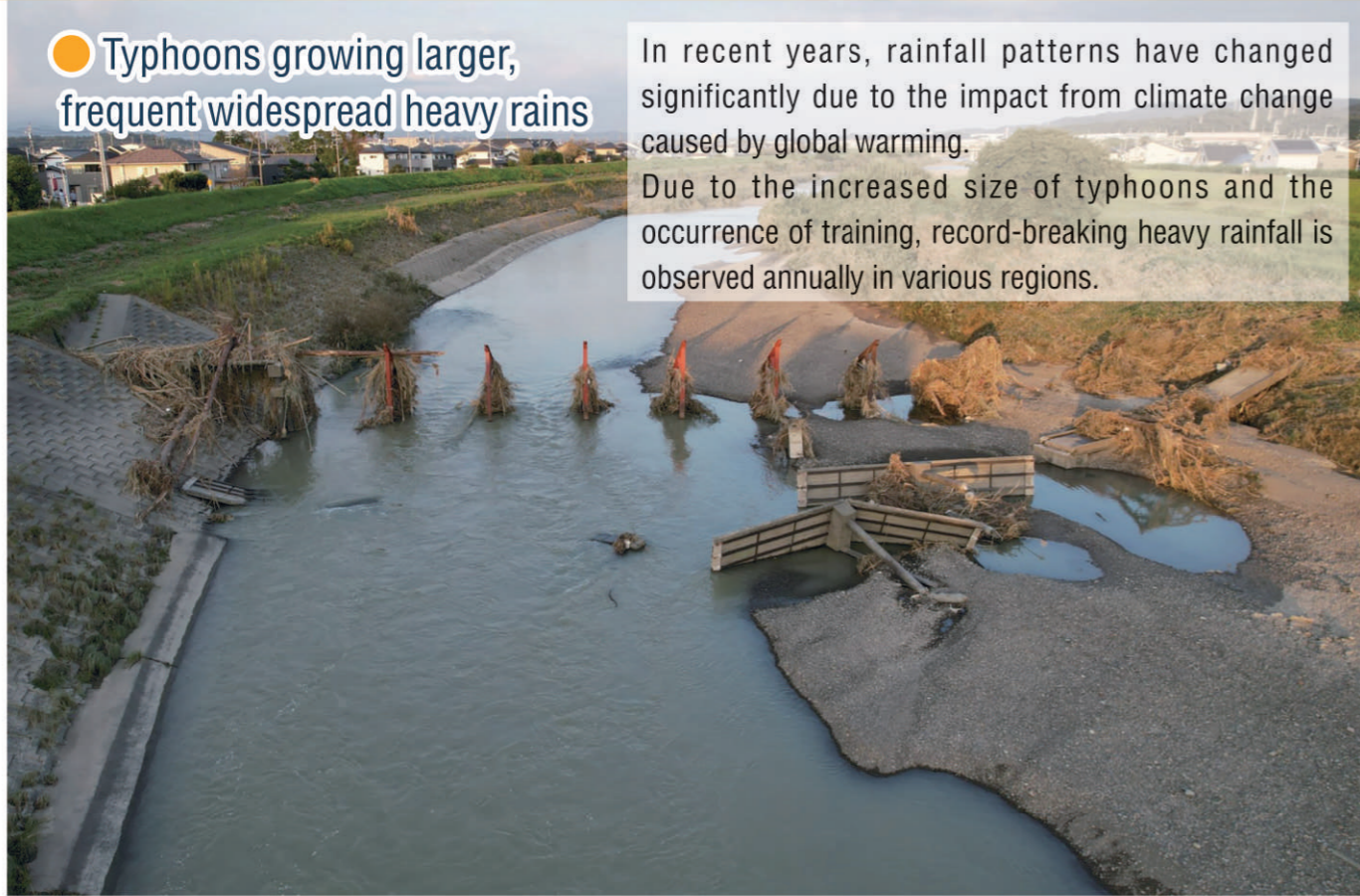
September 2022 Typhoon No. 15 Okano Bridge
