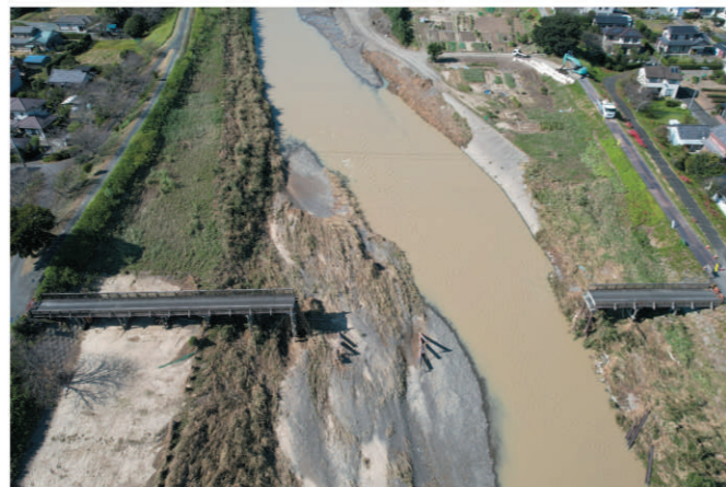
September 2022 Typhoon No. 15 Araya Bridge
