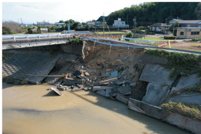
September 2022 Typhoon No. 15 Meiji Bridge
